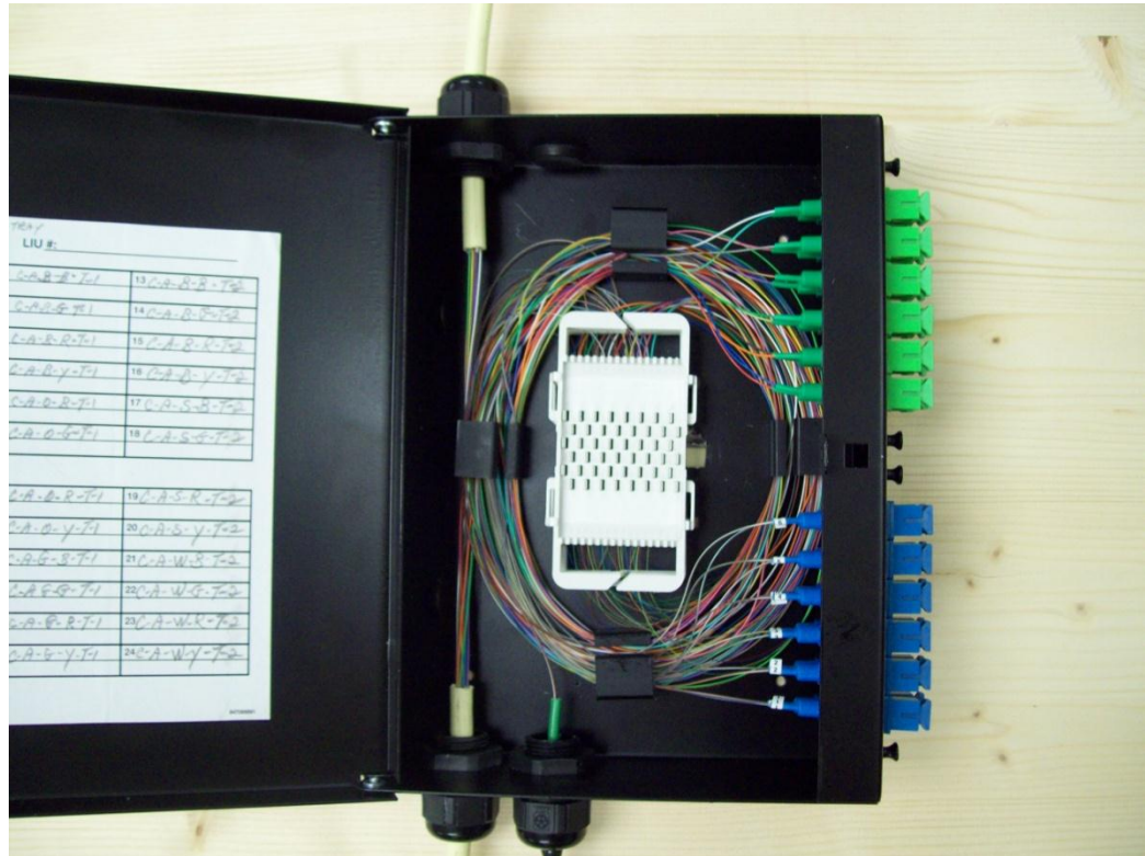
Figure 10 Pigtail Splice Installation
